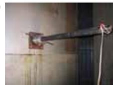
CARDOX tube is inserted in the tube holder and secured in the socket. Tube is then activated.
